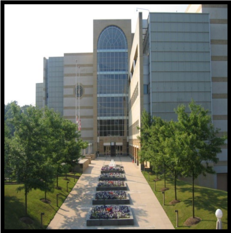
Southern Division Courthouse Greenbelt, Maryland
